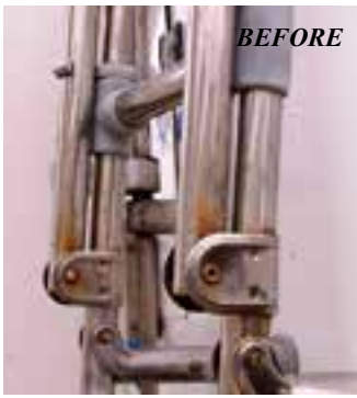
Rusty ladder cleaned with Super Stainless
